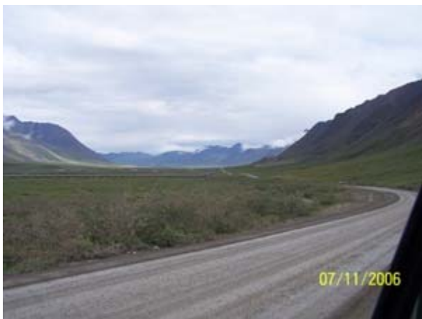
060711-22 Road down north side of Atigun Pass on Haul Rd
