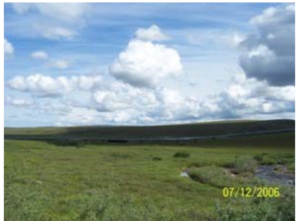
060712-19 Pipeline south of Prudhoe Bay
