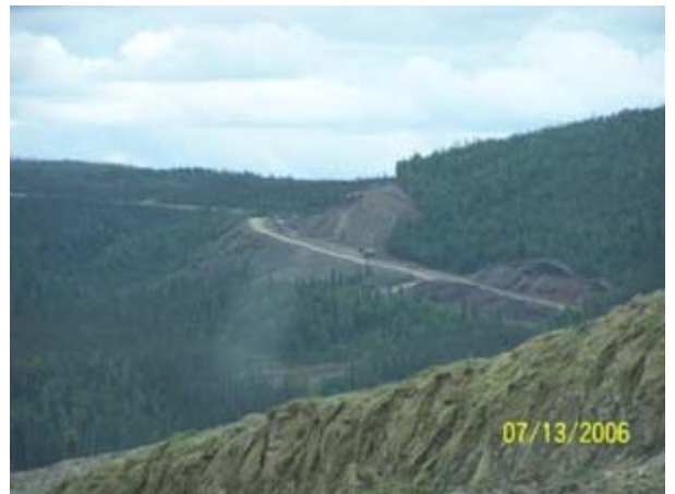
060713-03 Haul Rd construction
