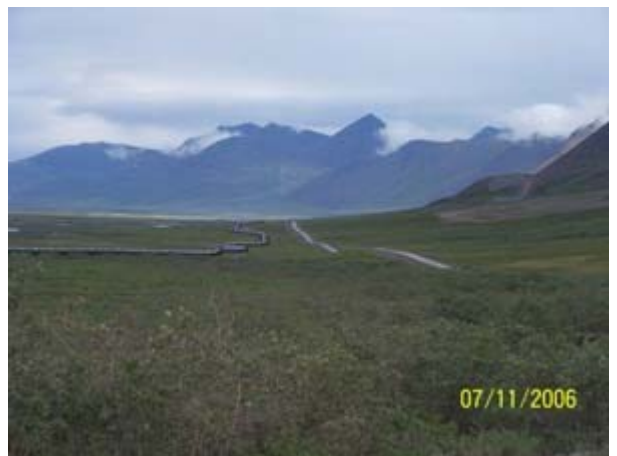
060711-23 Oil Pipeline & Haul Road
