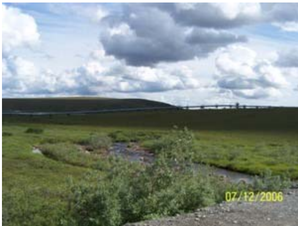
060712-18 Pipeline south of Prudhoe Bay
