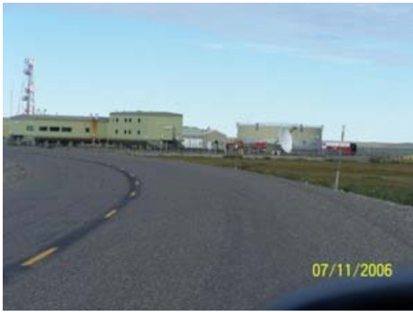
060711-40 Pipeline Pump Station 4 or 5
